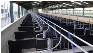
Covered finisher shed - would be considered fully enclosed
